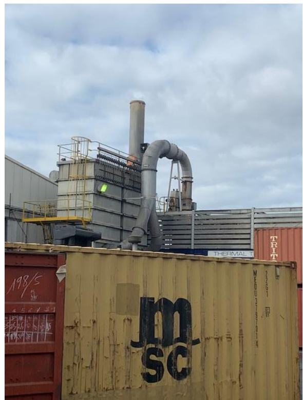
Photo 11 – Dust Collector & Stack TPP No 1
