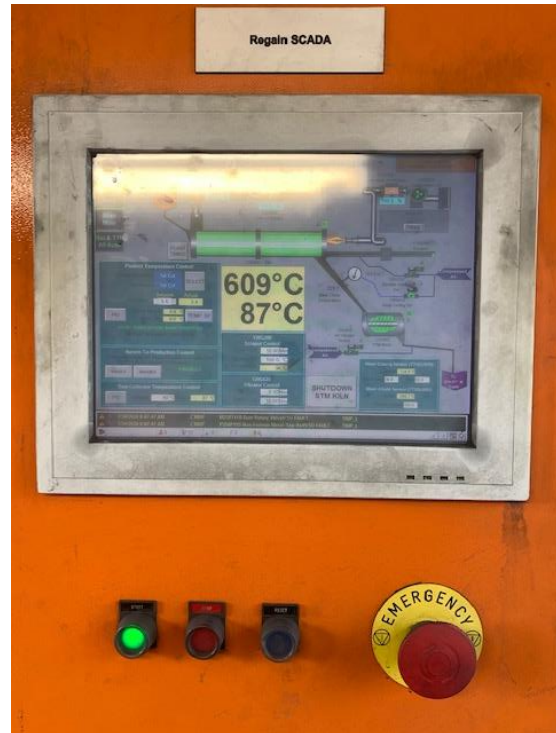
Photo 14 – SCADA SPL Thermal Treatment Plant 1
