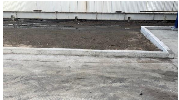
Photo 8 - Pavement Bunding
