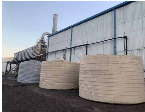
Photo 6 – Stormwater Storage Tanks - Upgrade
