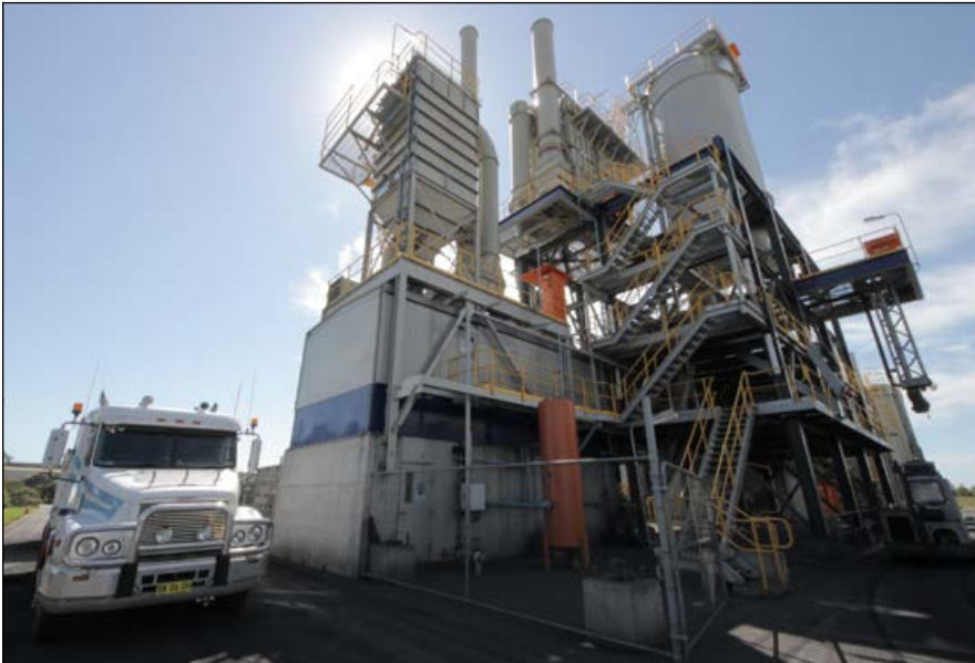
Figure 2. Innovative modular design by Regain is a major benefit in locating plants on-site.
