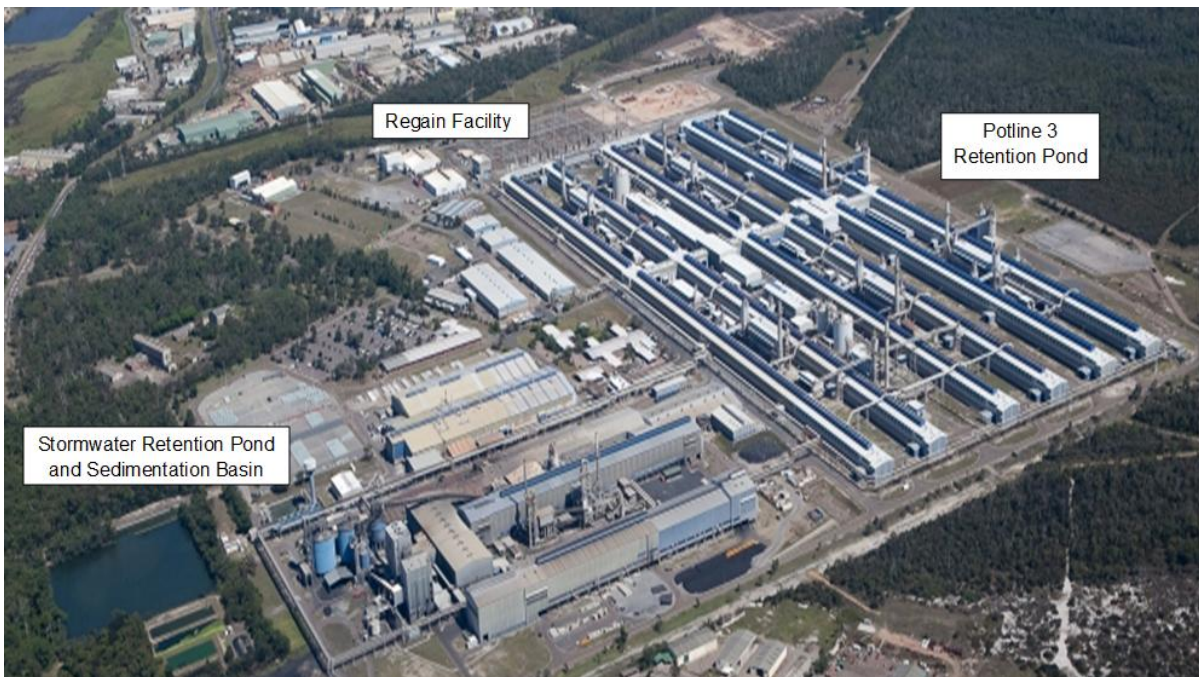
Figure 1 – Tomago Aluminium Site
